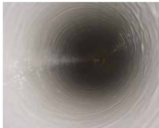
Before and after relining, using the Tomahawk pipe cleaning system in combination with a spray-in-place liner from 3M.
