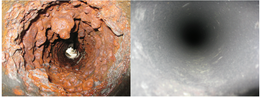
These photos represent the before and after images of a watermain cleaned with Envirolitics Engineering’s Tomahawk TR1 pipe-cleaning system. (Courtesy Envirolitics)
